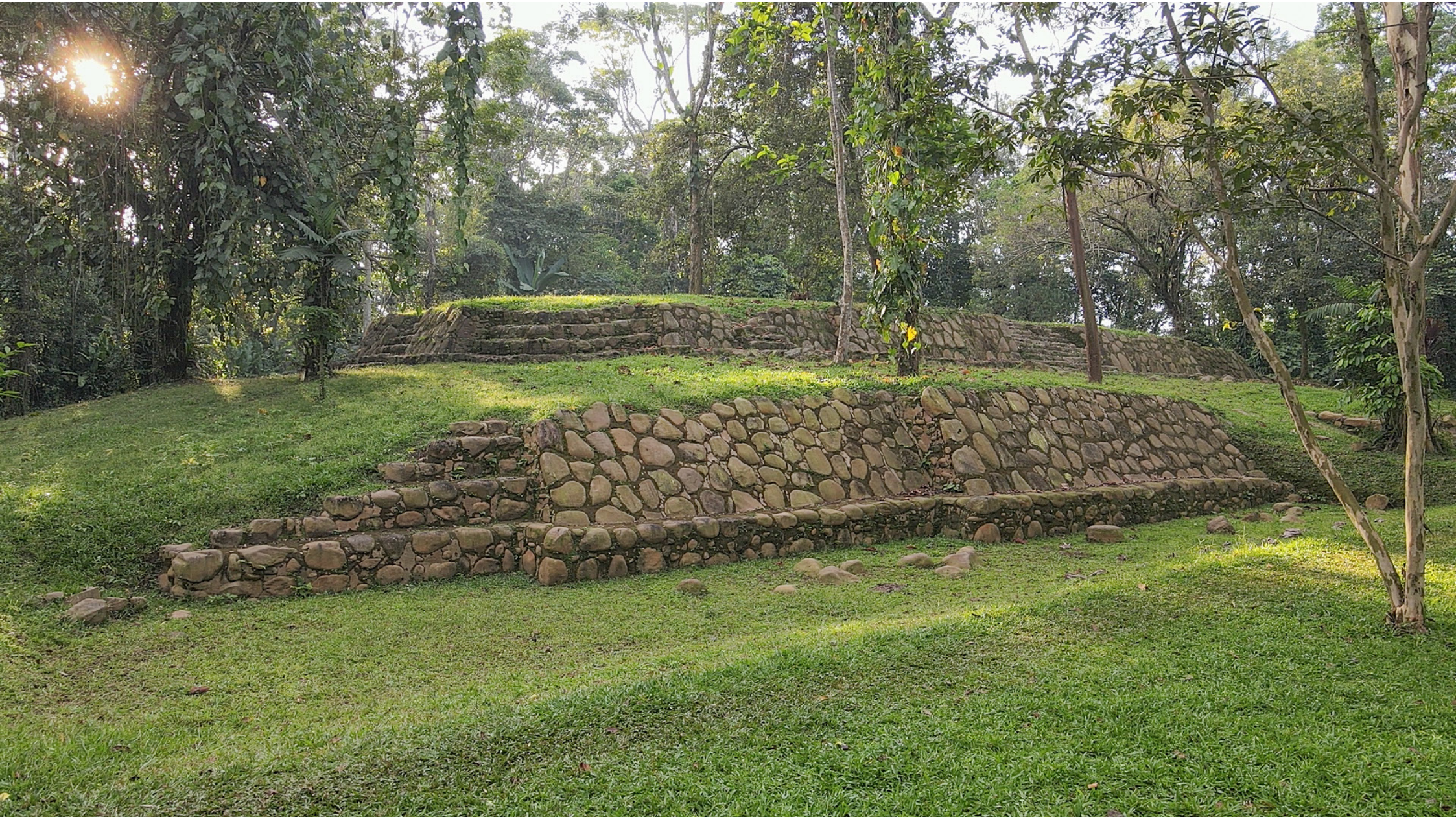
Fig. 59 Structure 6, terrace 3 with the characteristic regional constructive pattern
